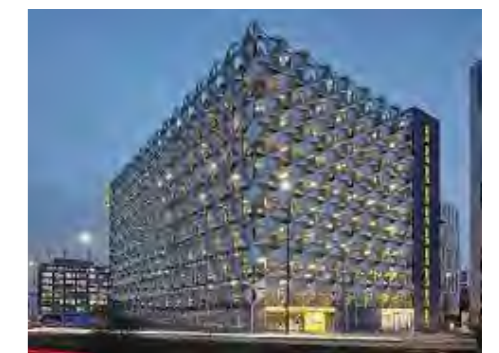
Stanley Street Car Park, Salford
